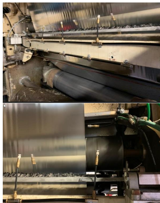
Figure 7. Dryer tunnel inlet pulverized water spray system.
