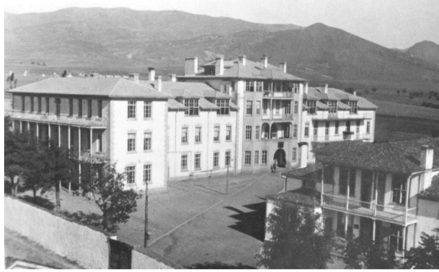
Figure 25. Anatolia College Hospital, 1900s, taken from the east. 28
