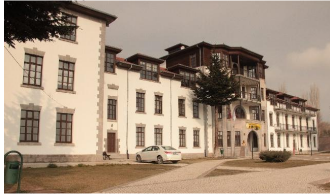
Figure 28. Anatolia College Hospital used as Merzifon High School for Science, taken from the east in 2019 (Gizem Özerol archive).
