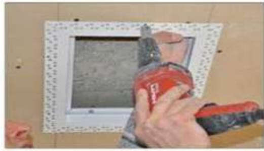
DIŞ ÇERÇEVE VIDALAMASI EN UÇLARDAN YAPILIR OUTER FRAME SCREWING IS MADE BY FASTENING SCREWS TO THE EXTREMITIES
